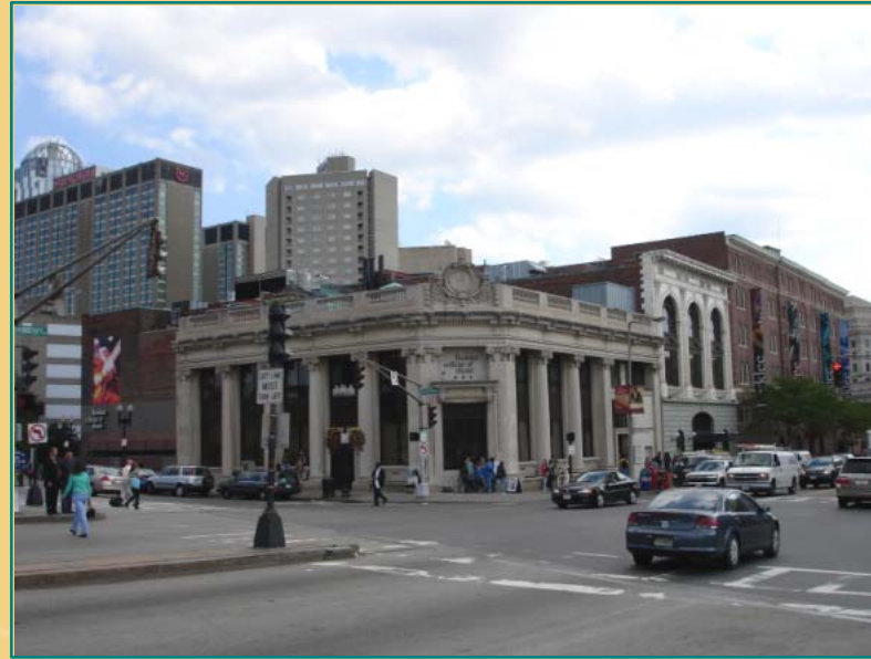
Corner of Massachusetts Avenue and Boylston Street
